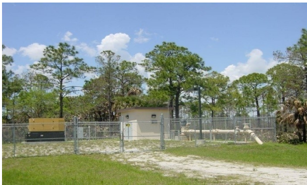
Photo 3. Production well building.
